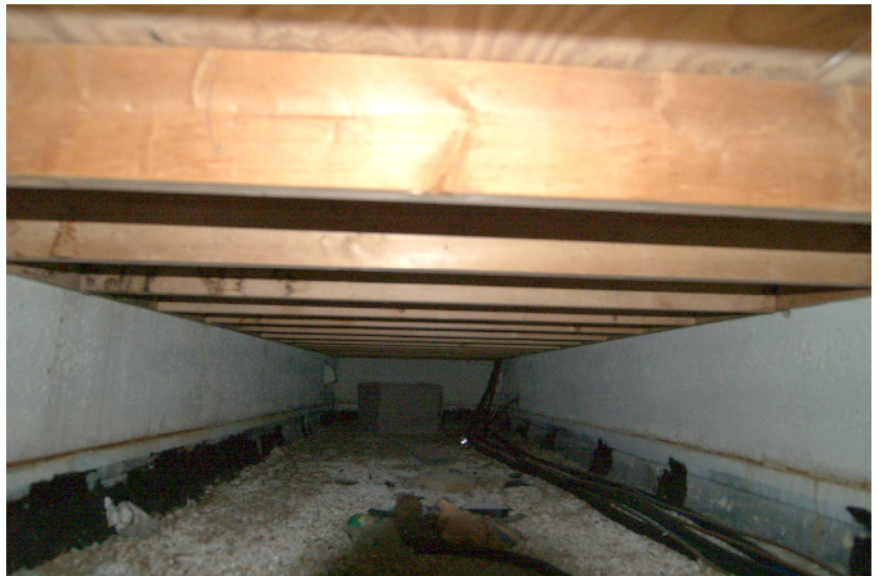
P021 Bluff Villas, Building 5 Right Side Lower flat roof section in front of A/C platforms. A few minor water leak stains evident on joist and plywood surface.
