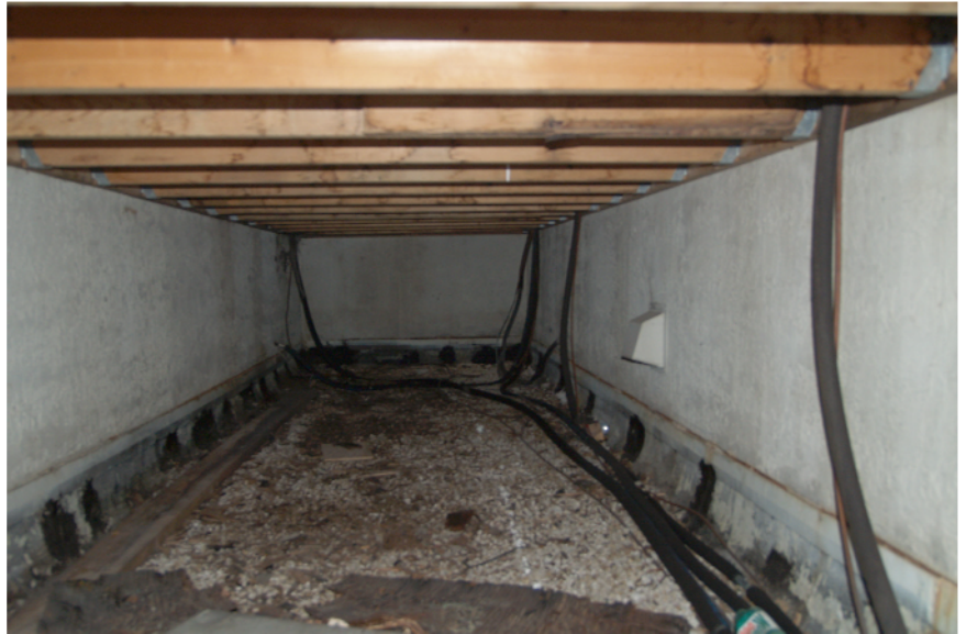
P020 Bluff Villas, Building 5 Right Side Upper flat roof section in front of A/C platform. Roof membrane separation evident at the joint.
