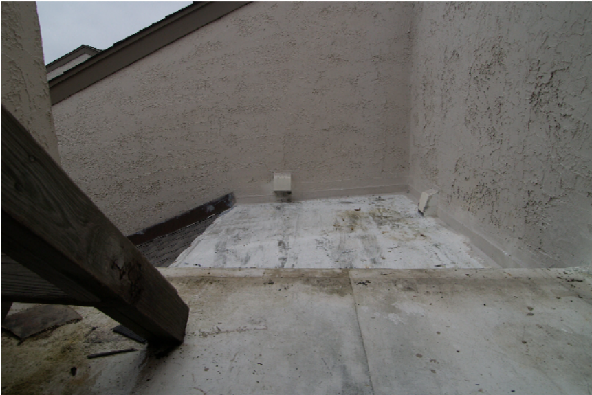
P021 Bluff Villas, Building 5 Right Side Lower flat roof section in front of A/C platforms. A few minor water leak stains evident on joist and plywood surface.
